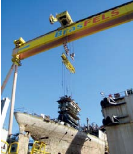
Keppel FELS Brasil's BrasFELS yard in Angra dos Reis lifting the last remaining Stork Hotlo diesel engine from the drillship Noble Roger Eason in support of a preservation project by a Dutch foundation
